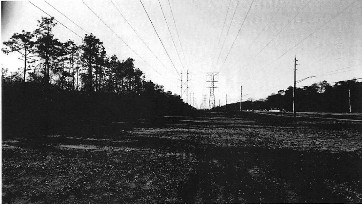
Subject Property Looking South Along Kernan Boulevard Source: Staff, Planning and Development Department Date: 02.03.17
